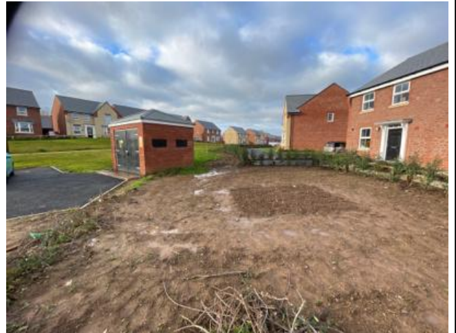
10. Pumping station at front, this may create noise during use, your legal advisor should confirm hours of operation and potential for disturbing you during occupation.
