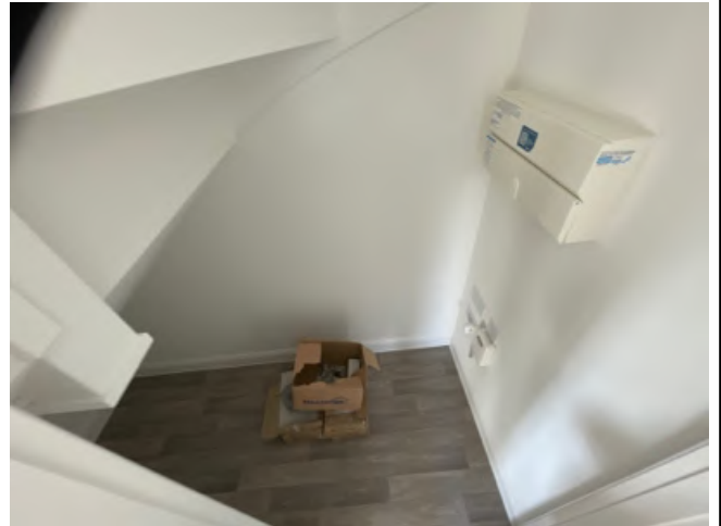
14. Ynder stairs cupboard
