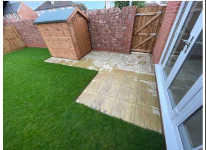
6. Rear garden patio. Timber shed cannot be opened as no lock installed.
