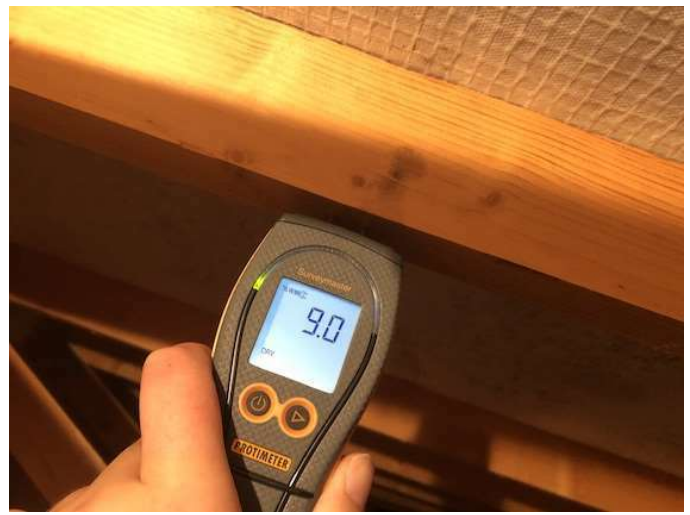
Roof damp meter reading
