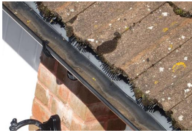
Gutter debris
