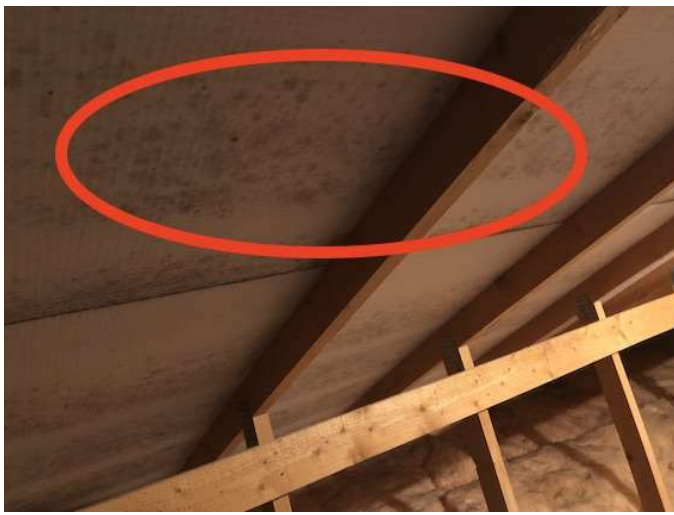
Underfelt mould
