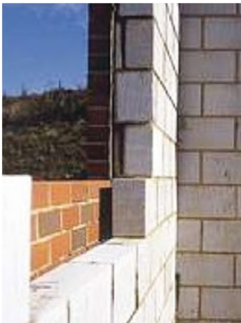
Fig1—Modern brick/block cavity wall
