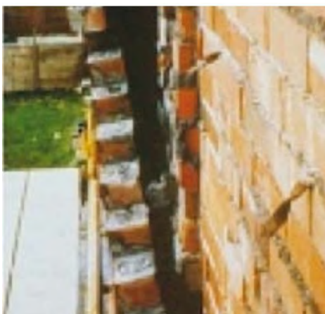
Fig5—Separation of outer leaf
