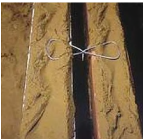
Fig2—Wall tie installation
