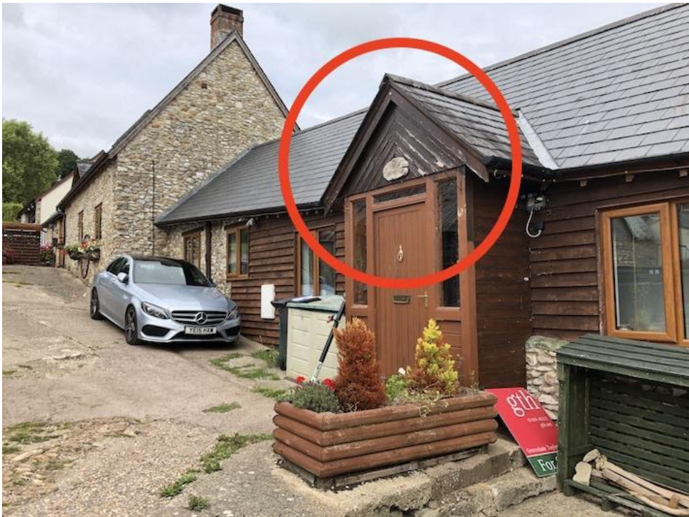
View of porch structure
