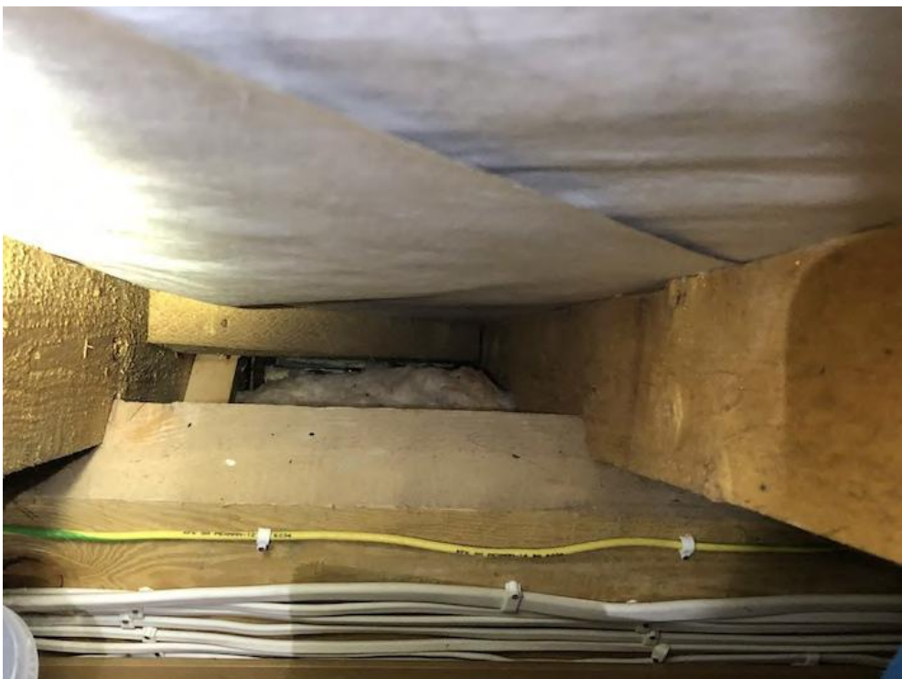
Purlin and underfelt
