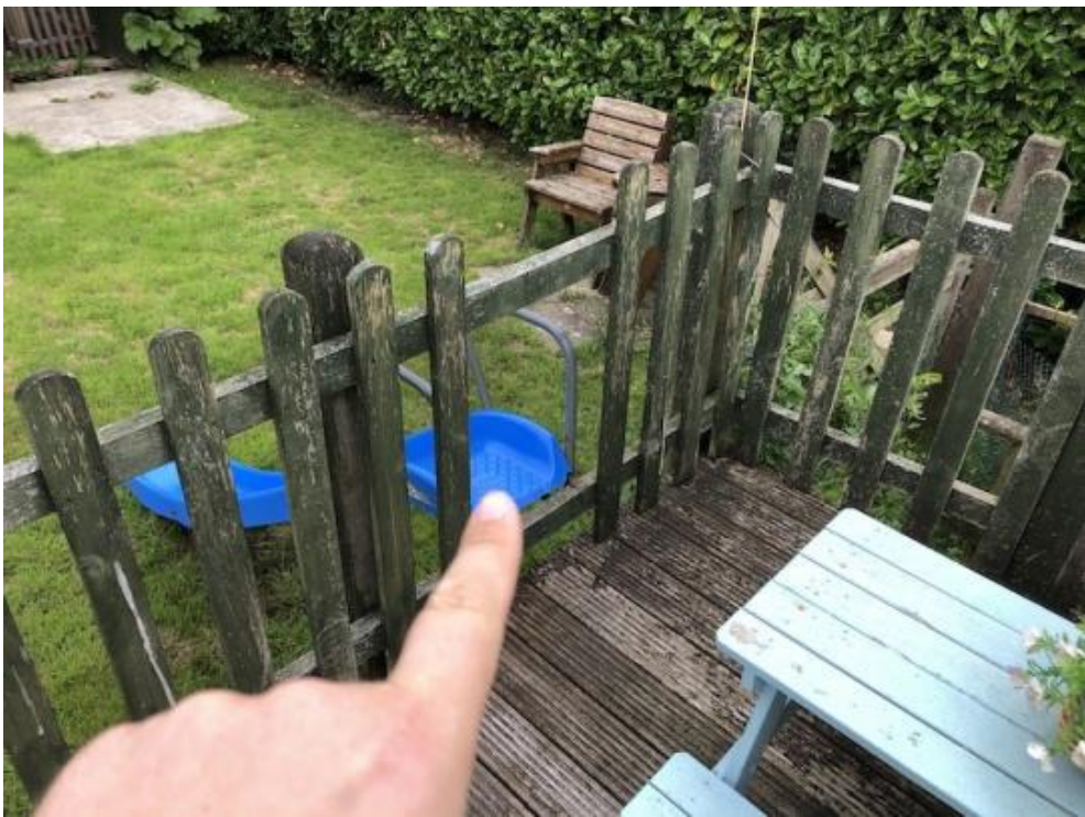
Decking fence hole
