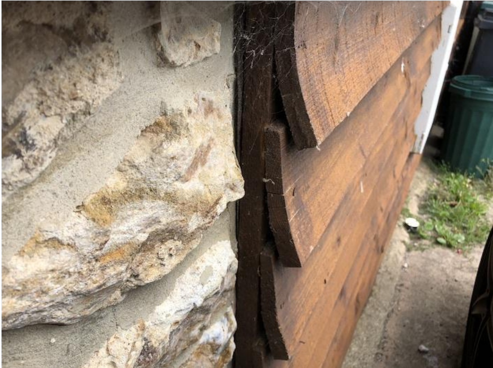
Timber cladding to front elevation
