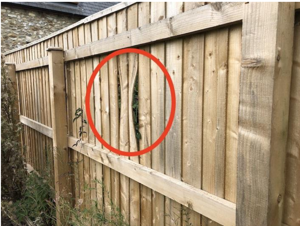
Rear left fence damaged
