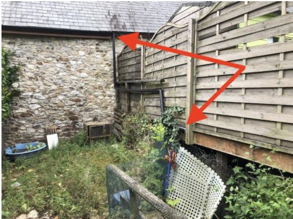
Rear right downpipe
